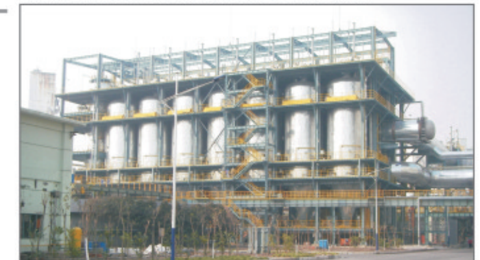
Primary dry dedusting system for 3x180t duplex converter of Chongqing Steel greenfield plant (EPC)
