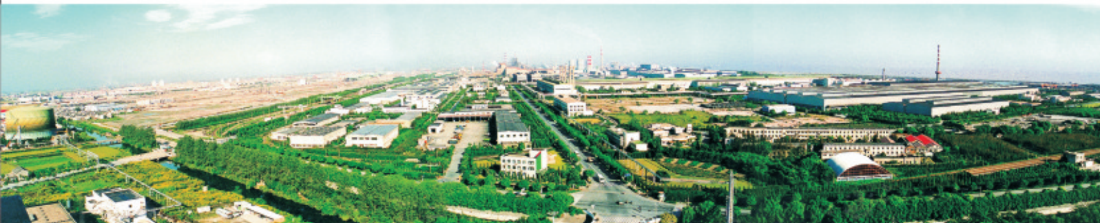
Baosteel – China's most modern large-sized iron & steel complex for which CISDI played as an engineering contractor
