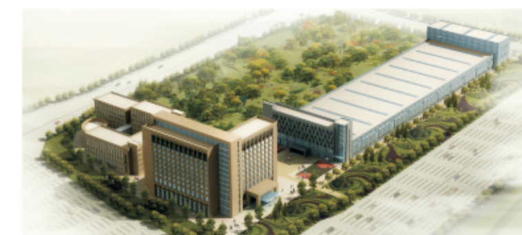
CISDI Electrical Base in Yizhuang, Beijing
