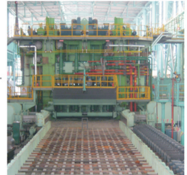
5000 mm Heavy Plate Mill of Shagang Group (Engineering)
