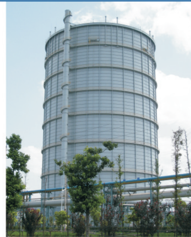
300,000m 3 Gas Holder in Baosteel (EPC), the first one in the world (pressure: 15kpa)
