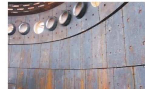
Cast iron/cast steel cooling stave
