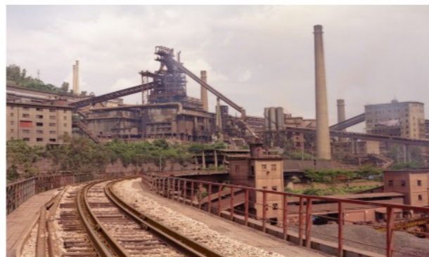
BF No.4 of PZH Steel Designed by CISDI
