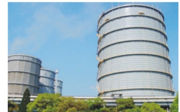
Baosteel 300, 000 m 3 Gas Holder Constructed by CISDI on EP Basis
