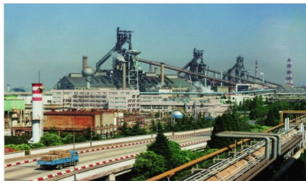
Series of BFs in Baosteel with volume over 4000 3 designed by CISDI
